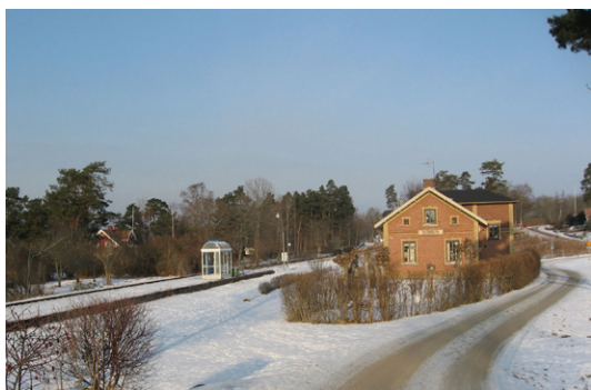
Blombergs station vintern 2012.
